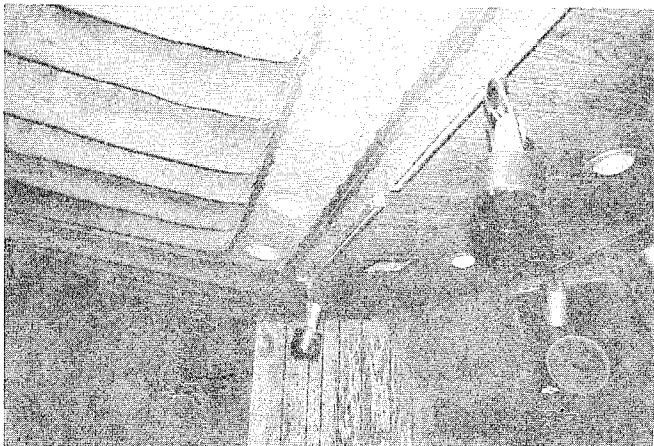
The absorptive front of the control room ends directly behind the console
