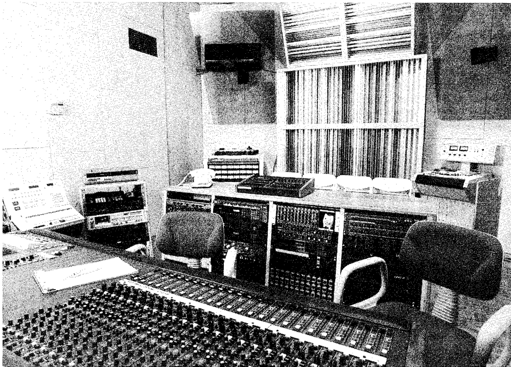
The control room rear wall has QRDs and PRDs and Haas Kickers.
